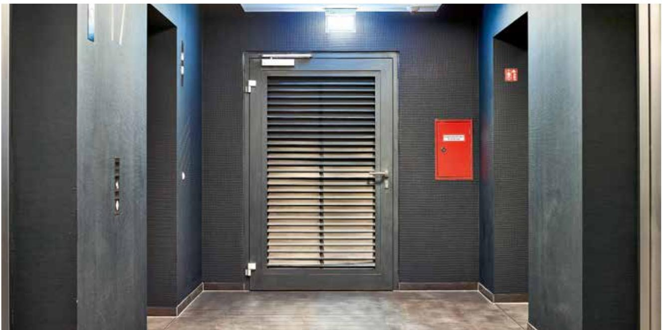
Opaque but not airtight: The custom-made product consists of a Hörmann tubular frame part and a mesh insert from Renson.
