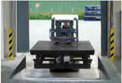
Position the new dock leveller
