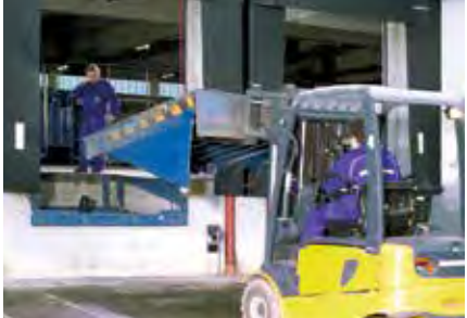
Remove old dock leveller, adjust pit if necessary (e.g. with fitting plates or support brackets)
