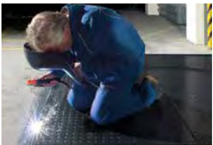
Weld to the edge brackets – done!
