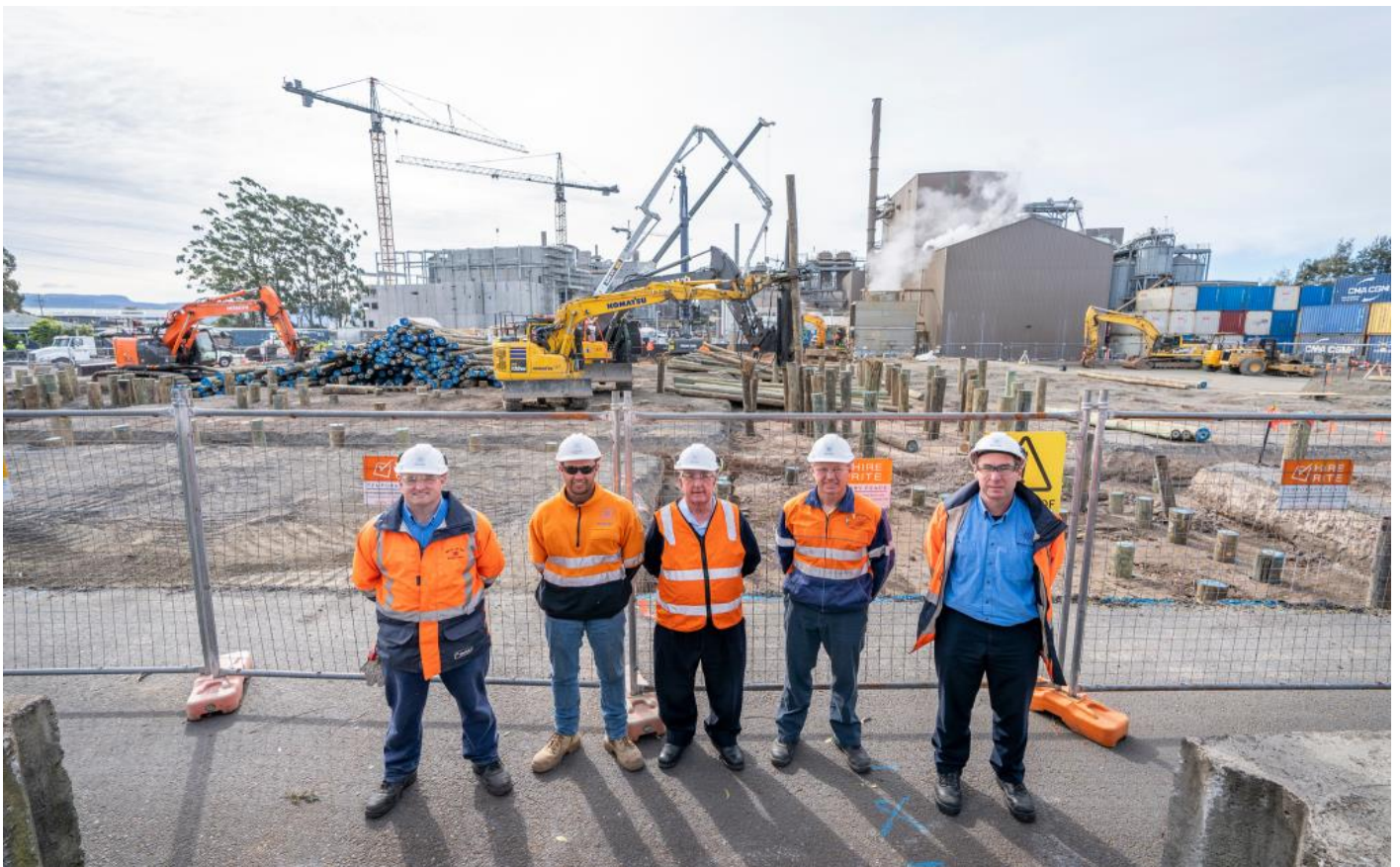
Manildra Group Breaking ground on Cogeneration Transition December 2022.
